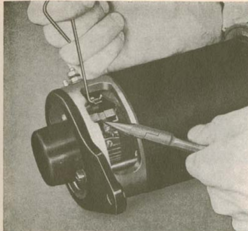
Fig. 10-34. Removing the brushes
