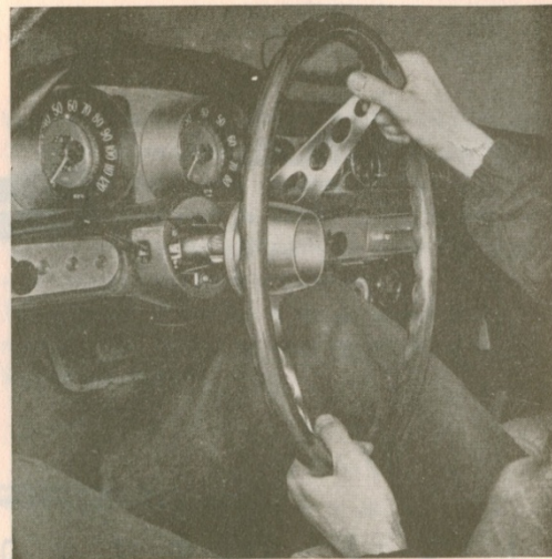
Fig. 6-21. Removing the steering wheel
